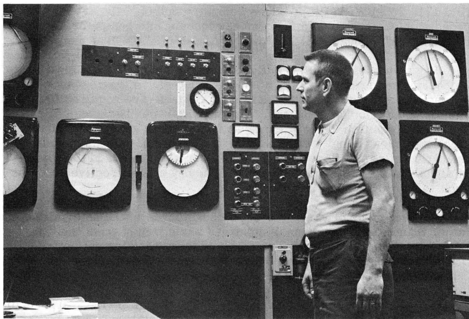
PRODUCTION FLOOR INSTRUMENT PANEL is used by Harding-Jones machine renders to determine process status.
