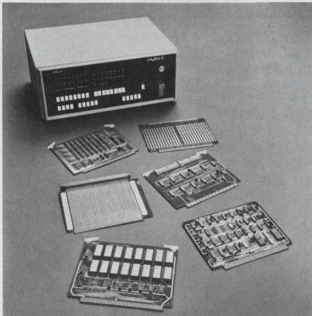
**Most manufacturers offer design aids** to simplify development of microcomputer systems. Intel's aids include the Intellec series, which comes complete with memory, supplies and clock and interface circuitry.
