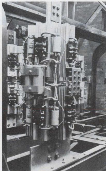
International Rectifier's diodes have replaced ignitrons in this caustic chlorine cell at Dow Chemical.
