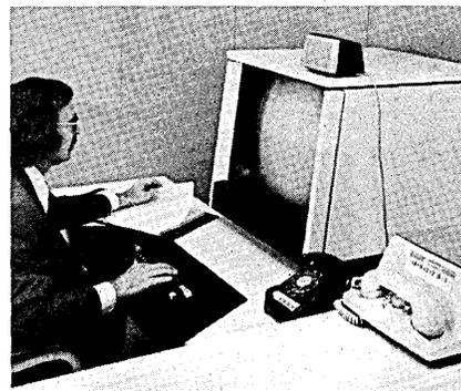
**DIAL A DIAGNOSIS:** From this mini-computer based console at Amdahl headquarters, computer engineers give instant maintenance back-up to firm's field engineers. It is used to scan out latches, examine machine status, run diagnostics, and even operates system using phone to link the customer's console with the Amdahl diagnostic assistance center.
