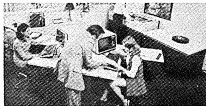
even easier to sell. (Singer claims an impressive 2,000 System Tens installed since late 1970.) All models use the same System Ten 6-bit processor with a 3.3 usec cycle time.
