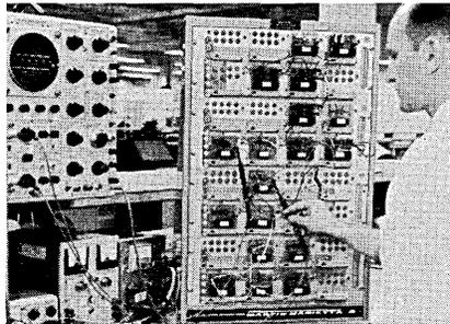
the design engineer a means of configuring various logic design schemes and enables him to see a logic diagram of the breadboard model. MARTIN CO., Baltimore 3, Md. For information:
