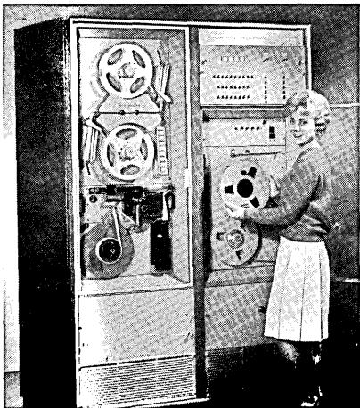
The device has a speed of 500 characters per second when operating in the magnetic tape mode. When converting data to paper tape, it has a speed of 250 characters per second. Five, six, seven, or eight-level paper tape codes can be accommodated, with or without parity. On the magnetic tape application, the converter operates with either the IBM 729 II/IV binary, or binary coded decimal low density format. Code translation, formating, and error-checking are performed automatically.
