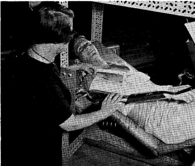
Figure 30. Myoelectric servo-booster arm-support sling.
