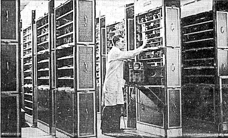
Fig. 6.3 The direct commercial descendant of the Cambridge EDSAC was a computer named LEO (Lyons Electronic Office) shown here in about 1953. LEO pioneered the use of computers for business data processing, as described further in Chapter 13.
