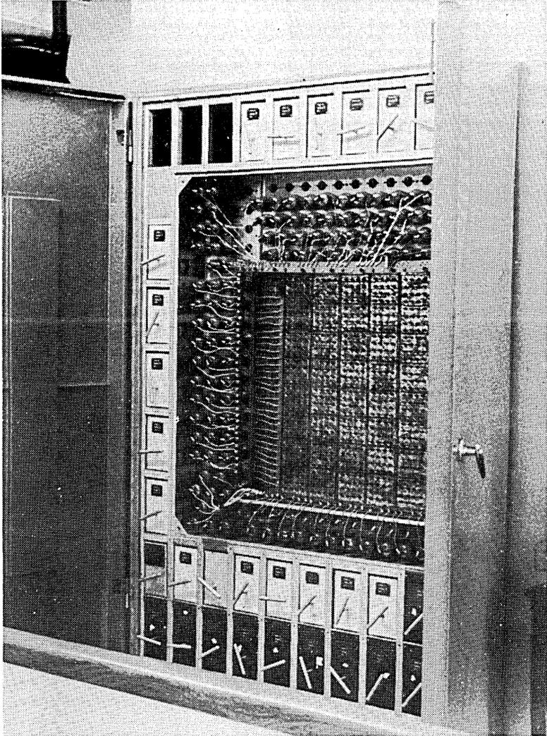
Fig. A1.6 A cabinet of the Cambridge University EDSAC II computer (1957), showing the microprogram control store. The important concept of microprogramming was first expounded by Professor Maurice Wilkes of Cambridge University in 1951.
