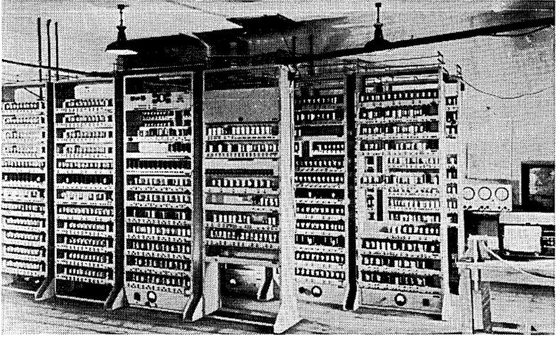
Fig. 6.2 The completed Cambridge EDSAC in 1949. This famous computer quickly settled down to provide an efficient computing service and helped to put Britain well ahead in the implementation of practical computers and their software.
